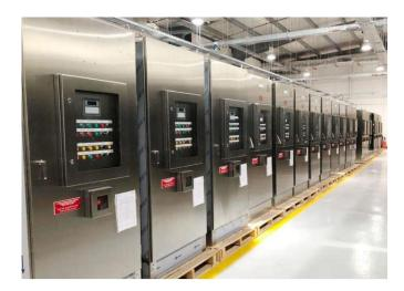
When designing a purge & pressurized system, purging multiple enclosures in series is an option that may arise when a single enclosure is impractical, for instance through overall size or potential problems with thermal management, or a complex piece of equipment requires separate interconnecting modules.
